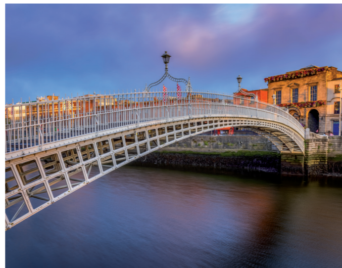
Ha'penny Bridge on the River Liffey, Dublin © Gareth McCormack – Ireland's Content Pool
